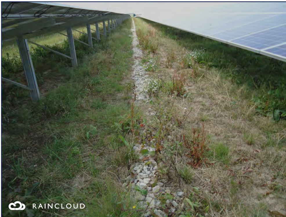
Plate A9.1.4320: Example filter drains at solar farms
